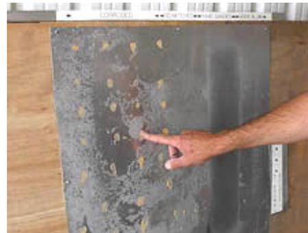
2. Work the surface in one direction only, typically from the top down. Slowly drag the pad down the surface at maybe 1” per second (or even more slowly) with the pad angled as shown in sketch. Use as much pressure as is reasonably possible.
